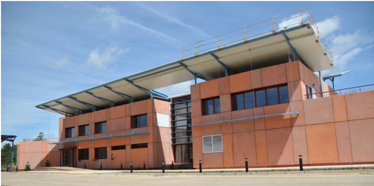
Figure 2 Demonstration building retrofitted by DRAGADOS (CEDER building, Cubo de la Solana, Soria)
