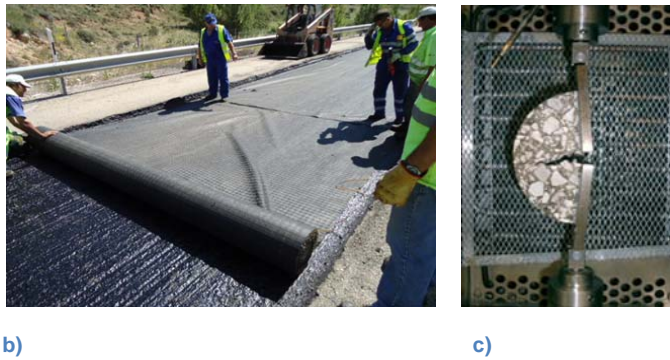
Figure 2 a) Deterioration models of semi rigid pavements. b) Reinforcement with geotextiles. c) Asphalt mixes resistant to reflection cracking and fatigue.
