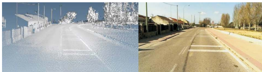
Figure 1 Three-dimensional scanning of an existing road
